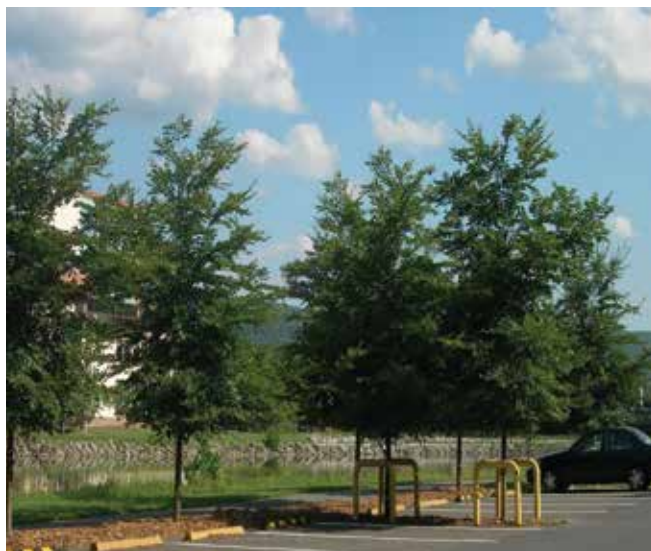
Figure 2. Parking lot design showing Accolade™ Elms planted in asphalt cutouts four years after installation. Trees are growing in a CU-Structural Soil® base with either nonporous or porous pavement on top.
