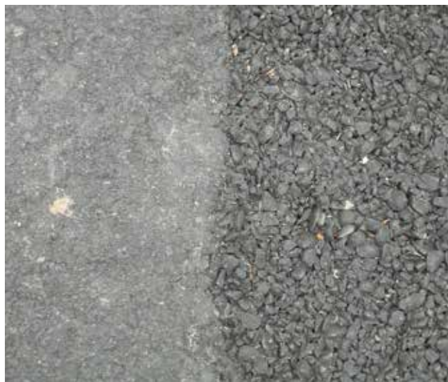
Figure 1. Interface between the nonporous (left) and porous (right) pavement in the parking lot installation.
