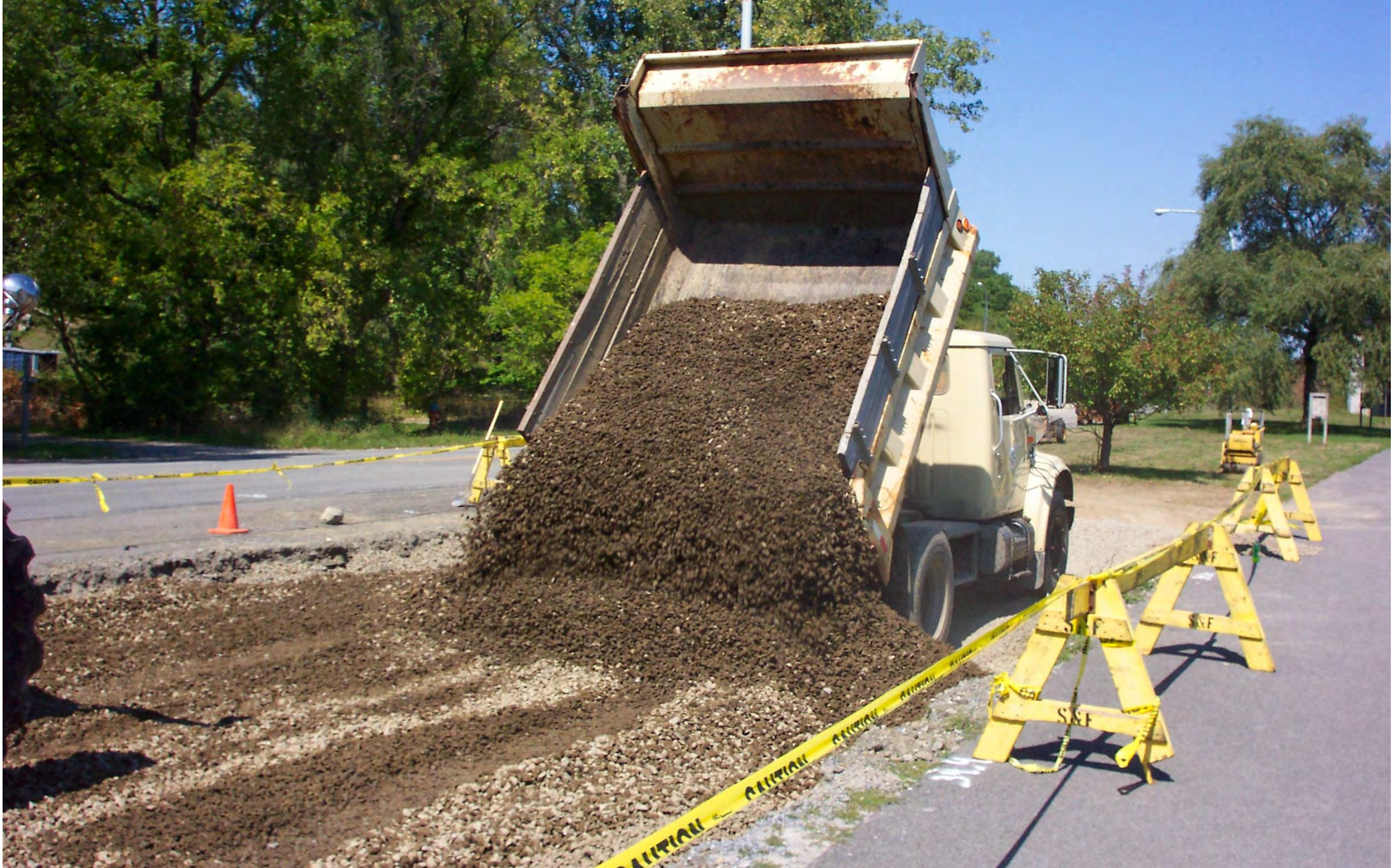
CU-Structural Soil® Parking Lot Installation – Ithaca, NY - 2005
