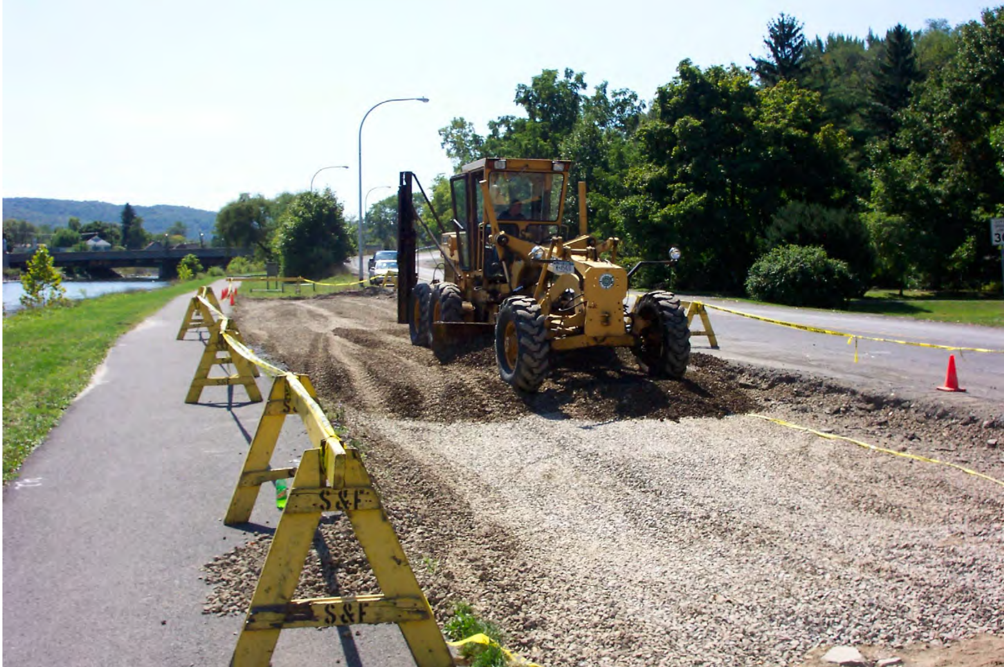
CU-Structural Soil® lift being graded prior to compaction
